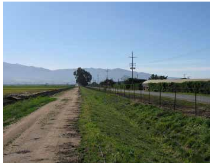
Native grasses were seeded; temporary upstream sediment trap was installed in winter to prevent siltation.
